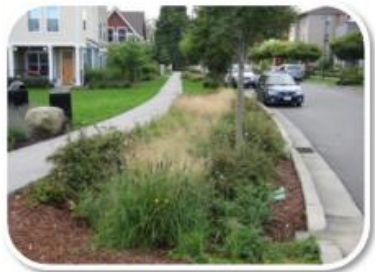
Bioswales and Rain Gardens
