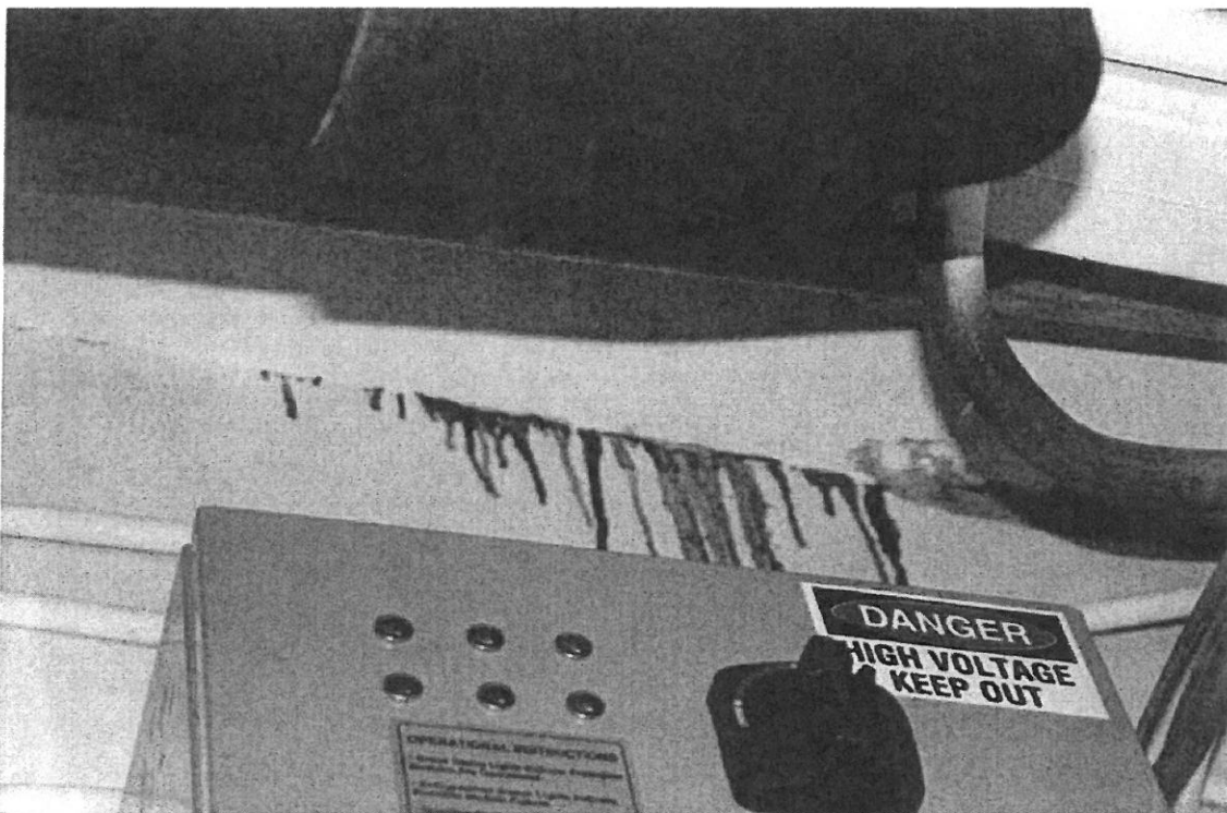
Repaired crack in wall, below water pipe and above electrical panel
