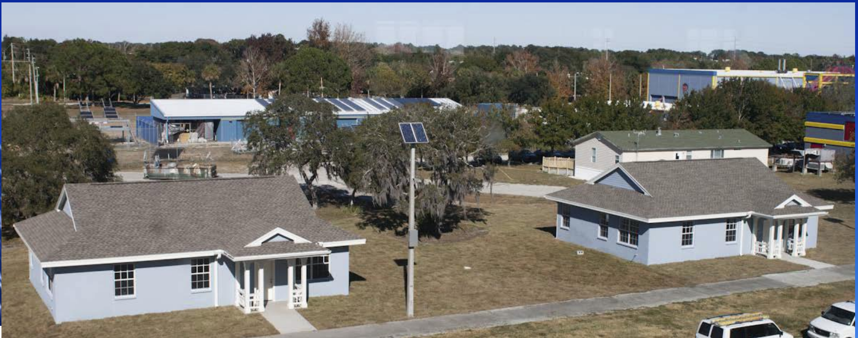
Flexible Residential Test Facility at FSEC
