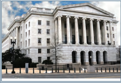
Longworth House Office Building
