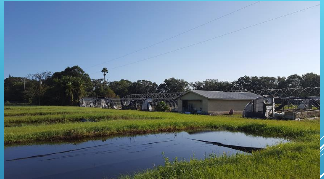
Flooding and Greenhouse damage, Plant City, Hillsborough County
