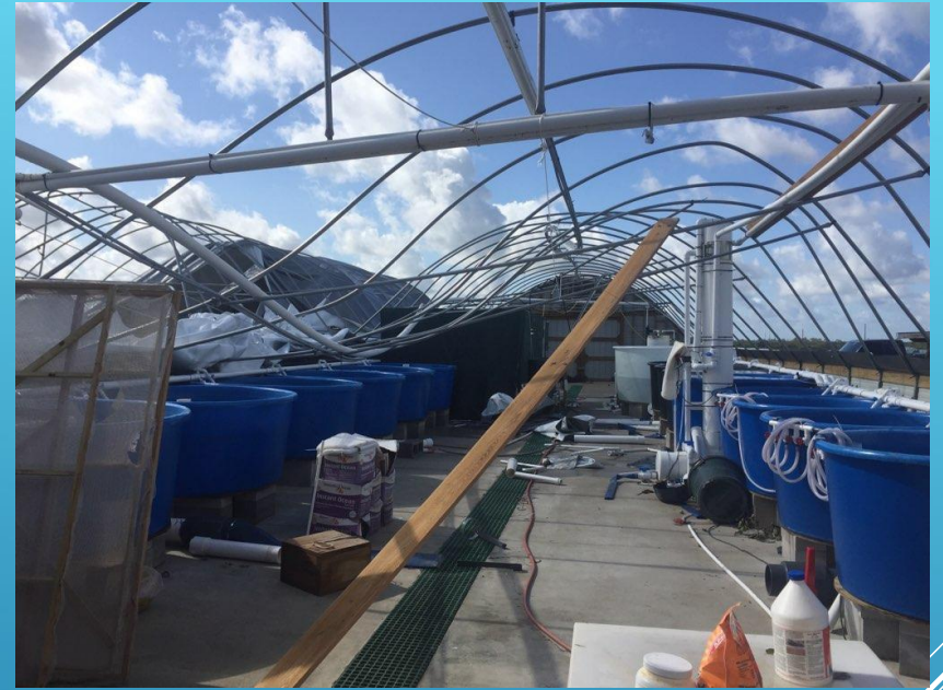
Pond covers and greenhouses destroyed, Arcadia, Desoto County
