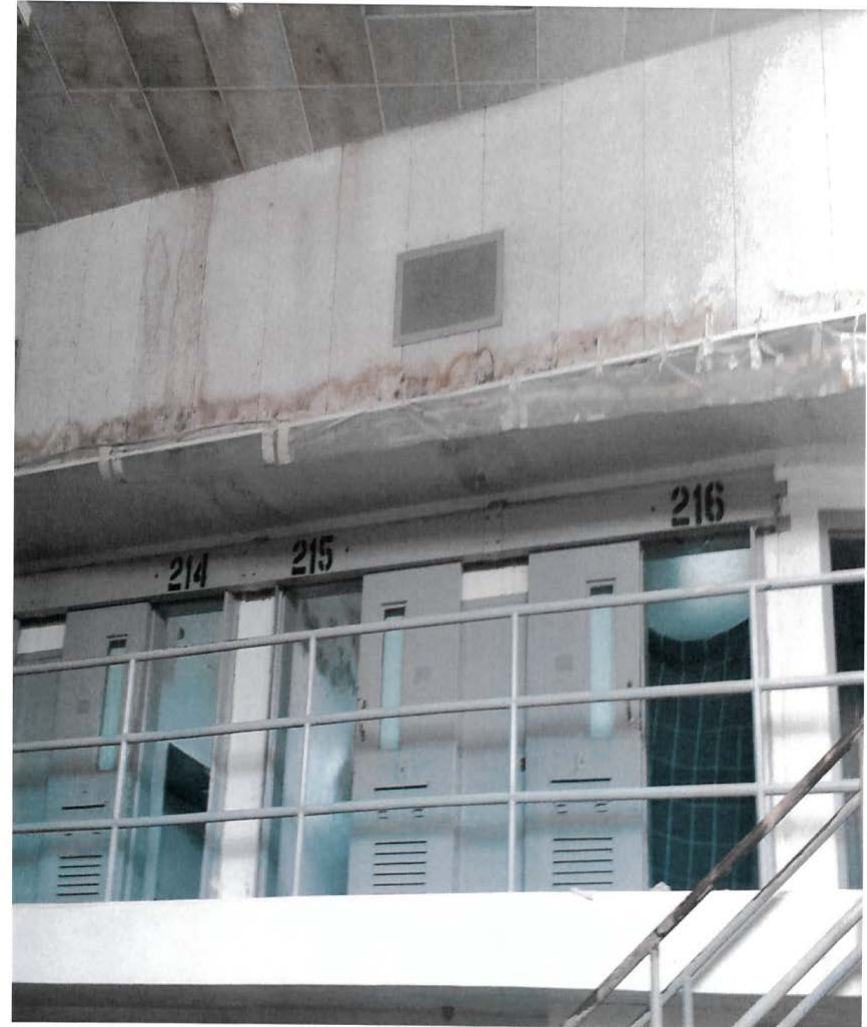
Examples of Leaking Roofs
