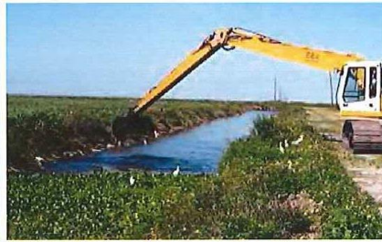
Systematic canal/ditch cleaning
