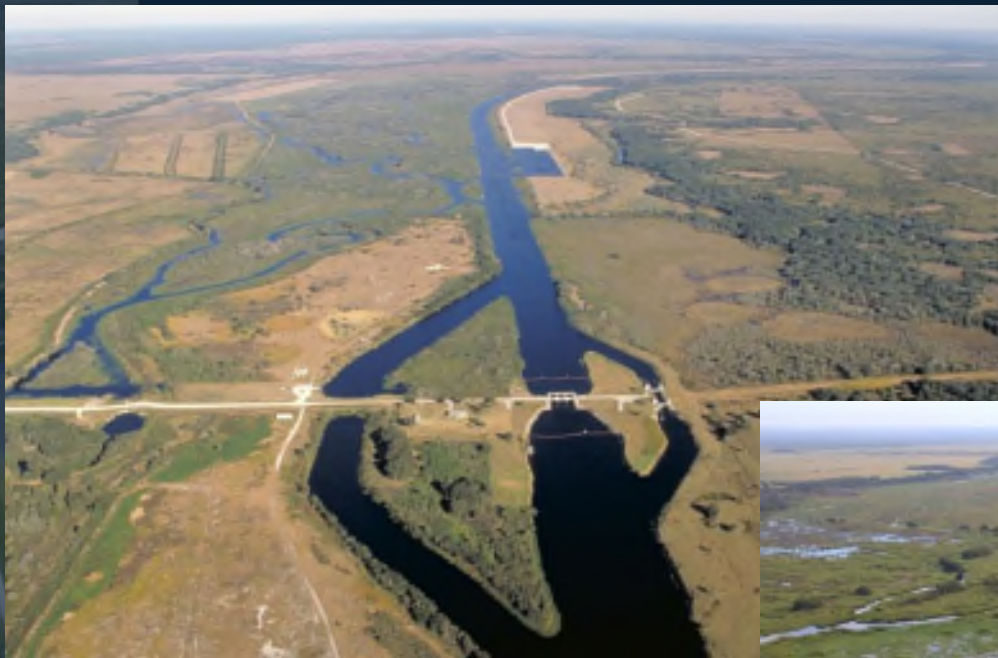
Kissimmee River Pre-Restoration Construction
