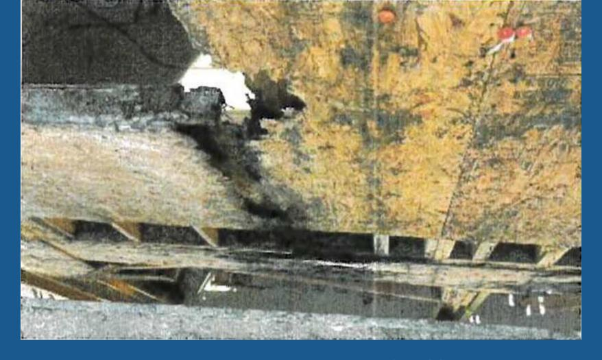
The water intrusion completely damaged the 2nd and 3rd floor OSB panels
