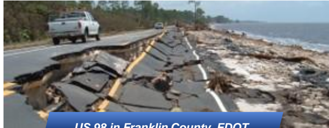
US 98 in Franklin County. FDOT
