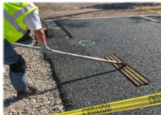
Pervious Pavement
