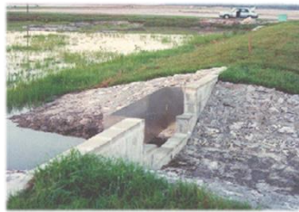
"Wet" Detention Ponds
