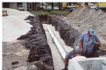
Underground Exfiltration Trenches
