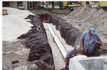
Underground Exfiltration Trenches
