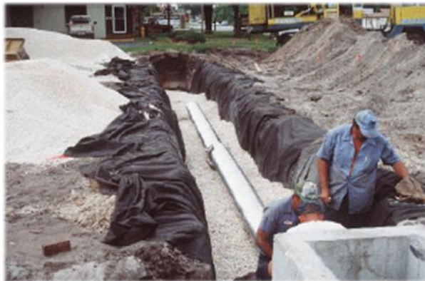
Underground Exfiltration Trenches
