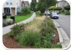
Bioswales and Rain Gardens • Improve property and neighborhood aesthetics • Reduce localized flooding • Promote infiltration and groundwater recharge • Enhance pedestrian safety when used in traffic calming applications
