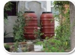
Rain Barrels and Cisterns • Reduce water consumption and associated costs • Reduce demand for potable water • Increase available water supply for other uses • Can significantly reduce stormwater discharges from roofs
