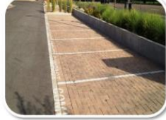
Permeable Pavements • Reduce stormwater runoff and standing water • Promote infiltration and groundwater recharge • Improve the longevity of infrastructure • May be easier to maintain than standard pavement
