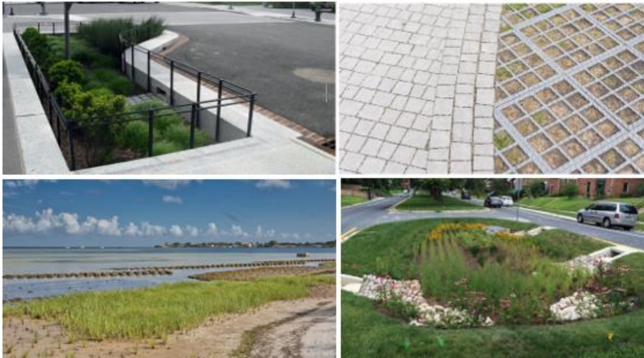
Stormwater Planter, Permeable Pavement, Living Shoreline, and Bioretention 9
